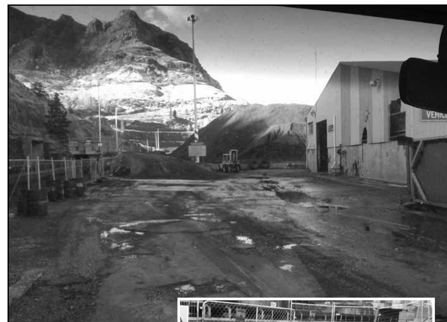
The vehicle workshop (inset) which was completely under water during the flood and where the runoff from the hillside comes under the coal conveyor belt and pours into the vehicle workshop yard.
