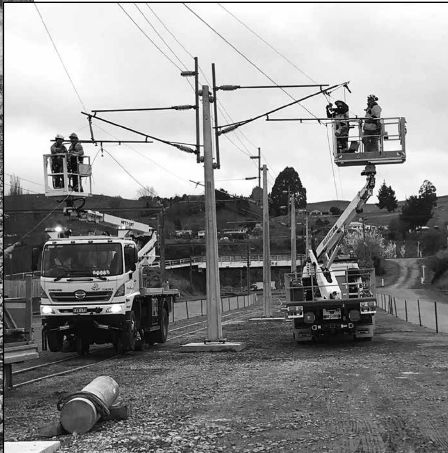
(below) Setting up overhead wires ready for the new EF locos.
